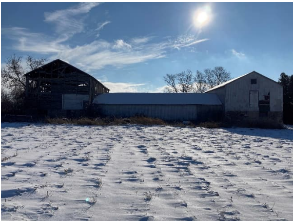
Plate 90: West elevation of complex showing connecting shed
