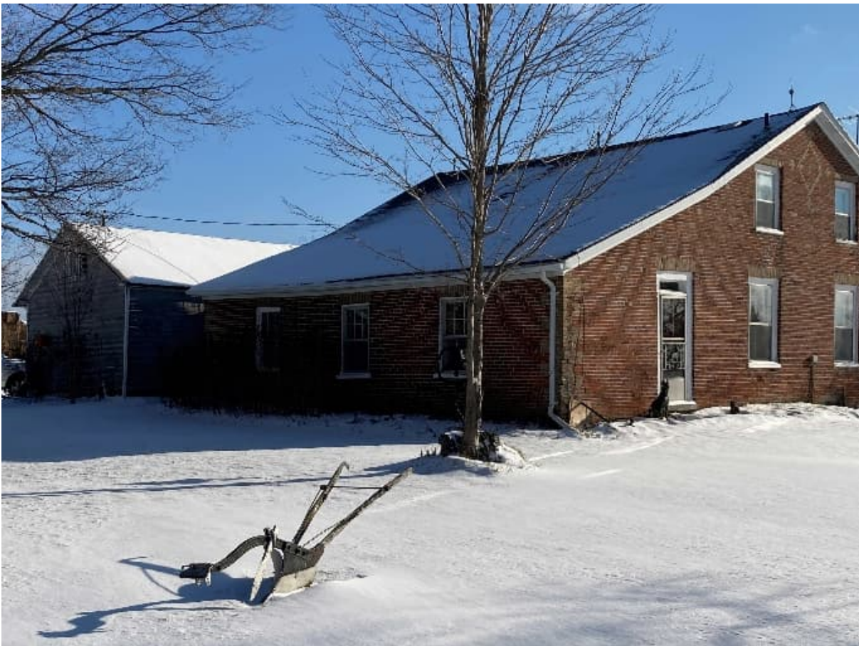
Plate 64: Oblique view of side addition
