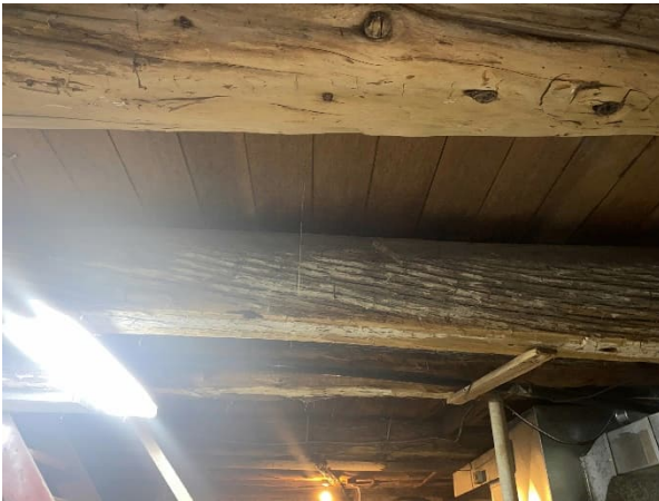
Plate 35: Hand hewn log floor joists
