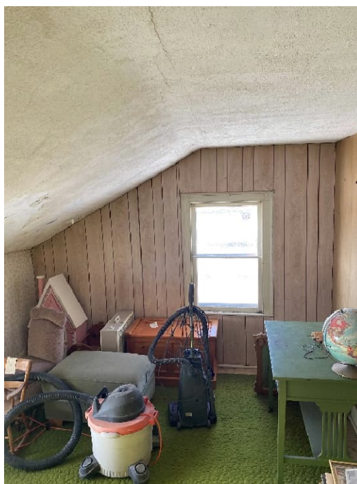
Plate 49: Southeast room of second floor
