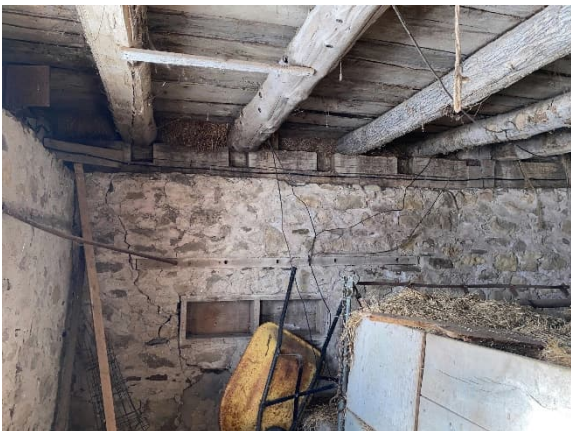
Plate 98: South barn interior, redundant mortices visible along sill
