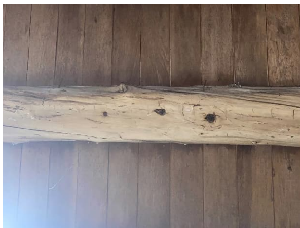
Plate 37: Main block plank subflooring
