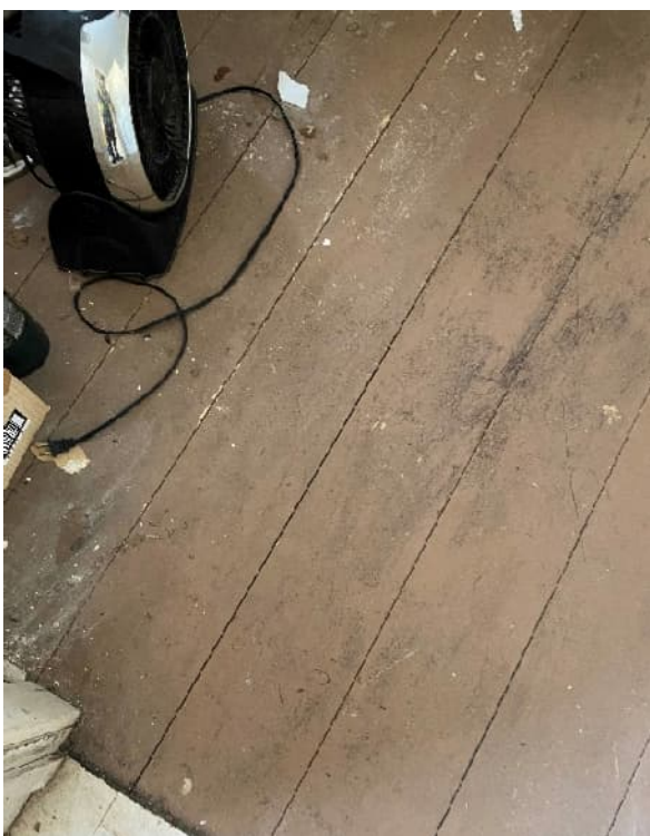
Plate 73: Wood floors of Rear addition storage room
