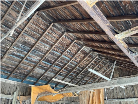
Plate 102: Interior of Outbuilding No. 1 showing rafters and plank sheathing of the roof
