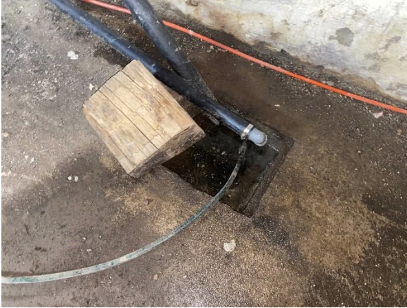
Plate 33: Poured concrete basement flooring
