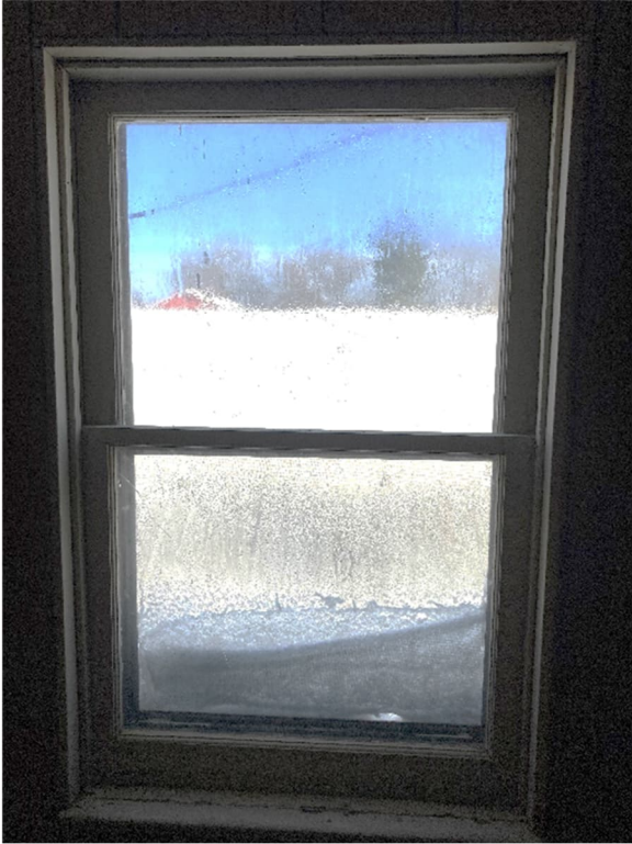
Plate 61: Detail of north window
