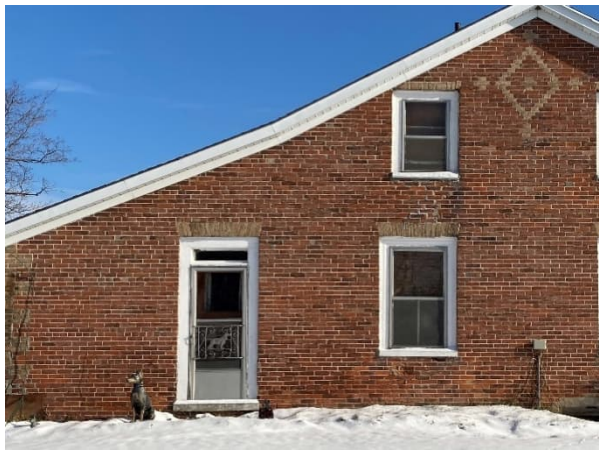
Plate 23: Limit of main block (right) and rear addition (left)
