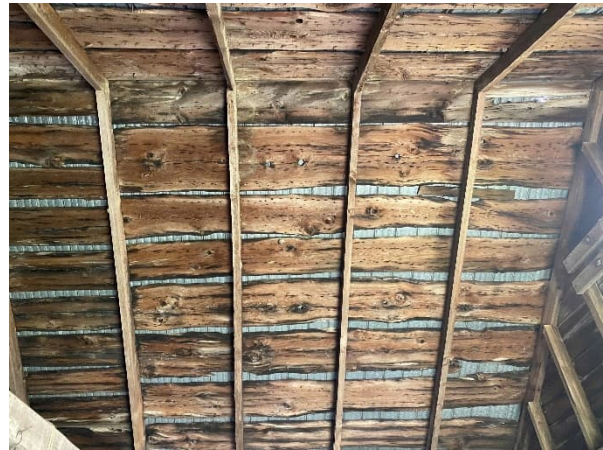
Plate 87: Wide board roof sheathing
