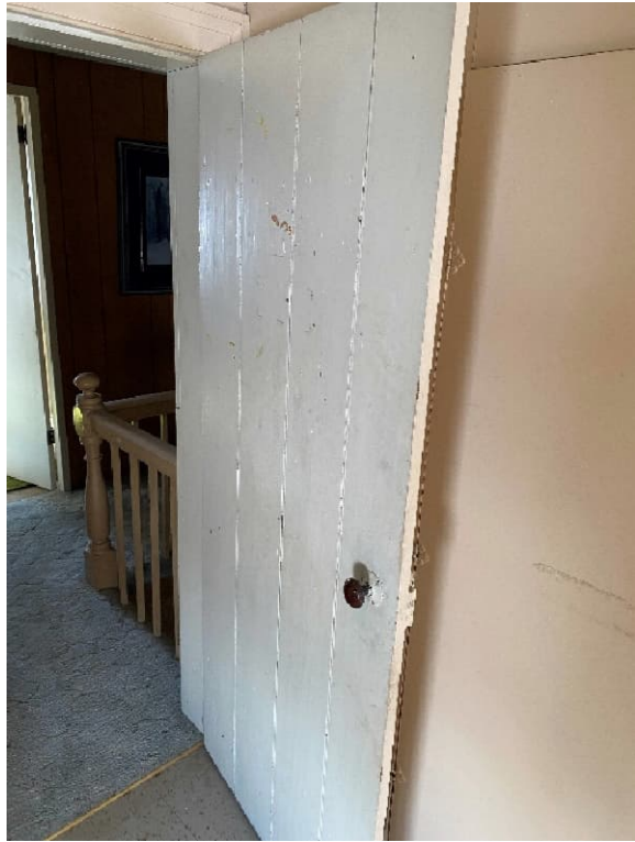
Plate 57: Vertical panel door to northeast room
