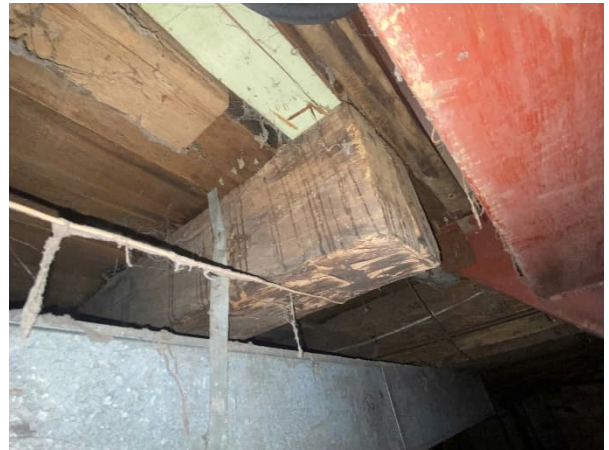
Plate 36: Hand squared floor joist
