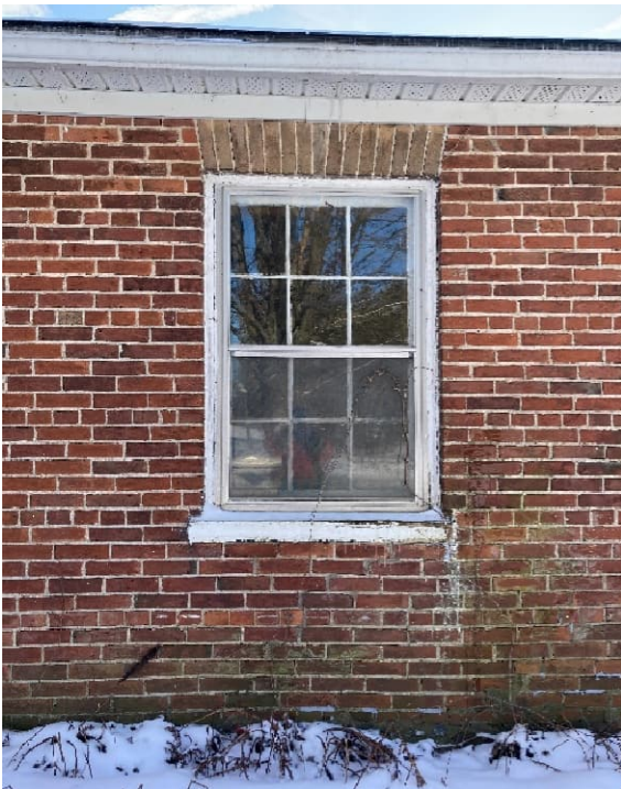
Plate 67: West elevation window
