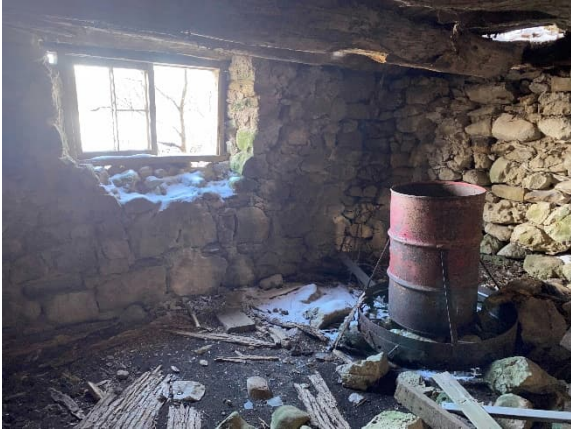
Plate 94: North barn interior showing rubble stone foundations
