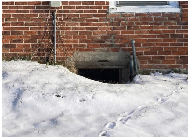
Plate 21: South elevation basement window
