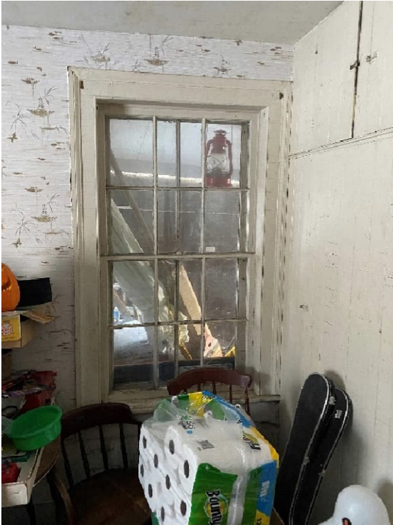
Plate 75: North elevation window into side passage
