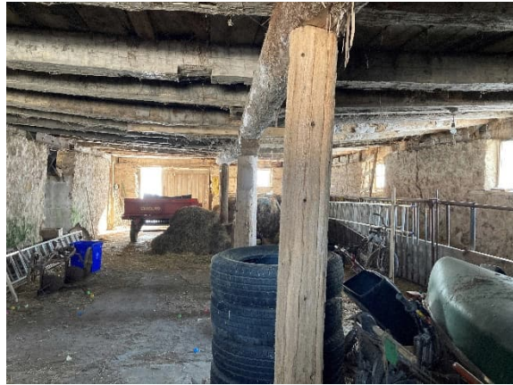
Plate 97: South barn interior showing hand hewn beams and redundant mortices
