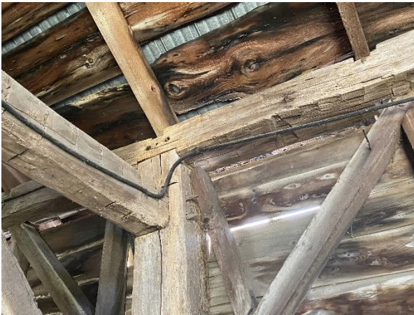
Plate 86: Mortise and tenon timber joints with wood treenails/dowels
