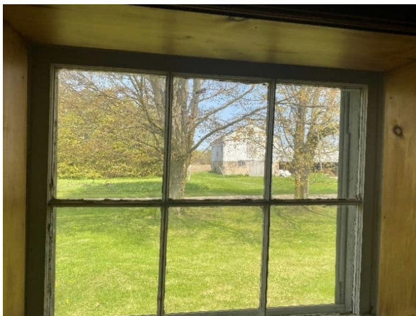
Plate 71: West elevation window
