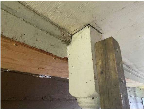
Plate 79: Original veranda pillar
