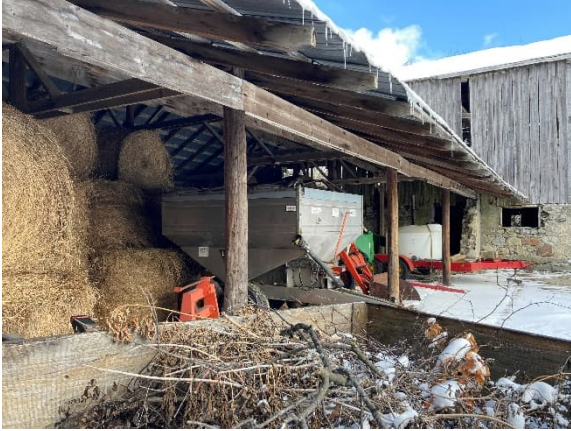
Plate 100: Junction between connecting shed and north barn
