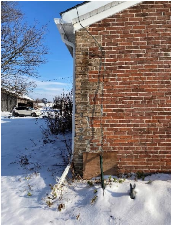
Plate 65: Detail of southwest corner, showing quoins
