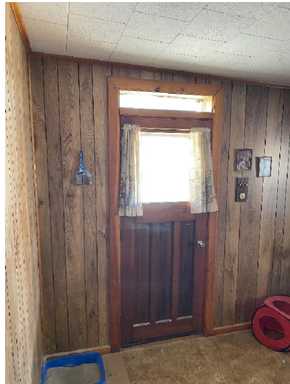
Plate 70: South entrance to rear addition
