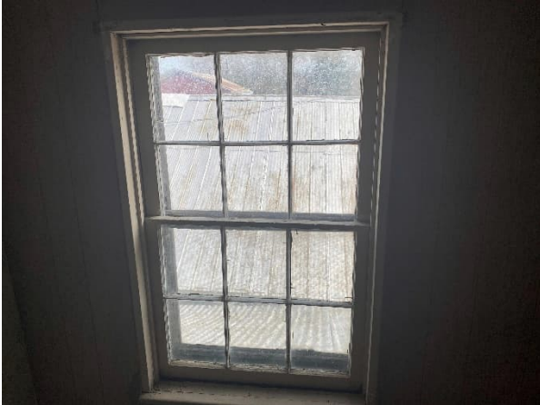
Plate 52: Six-over-six sash window in northeast bedroom
