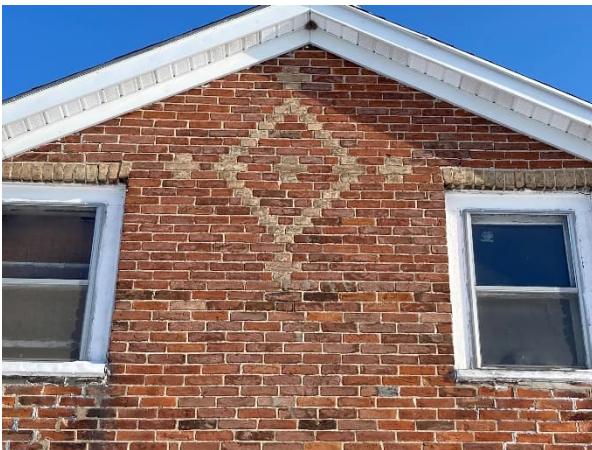
Plate 22: Buff brick diamond and cross pattern
