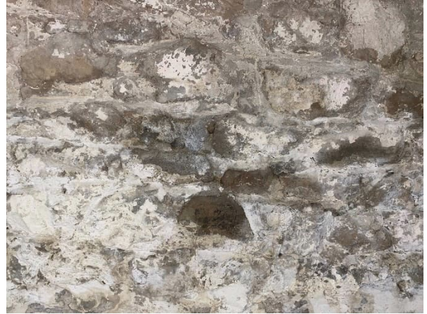
Plate 34: Parged stone foundation
