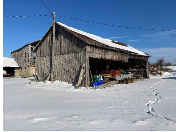
Plate 101: Outbuilding No. 1 (timber framed drive shed)
