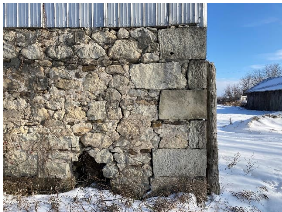
Plate 93: Foundation and cut stone cornerstones of south barn
