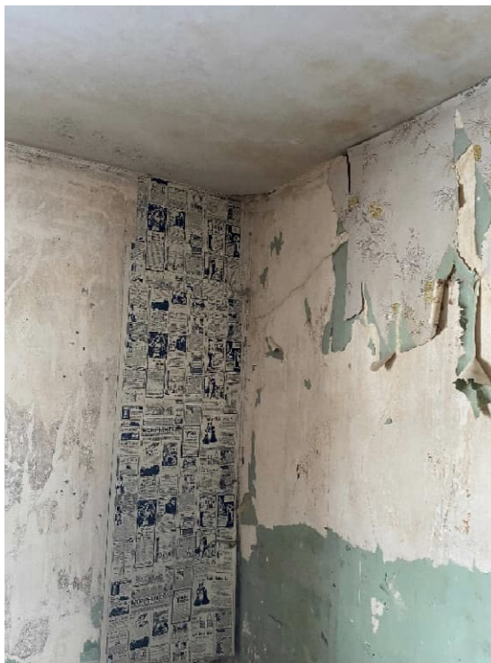
Plate 72: Rear addition storage room
