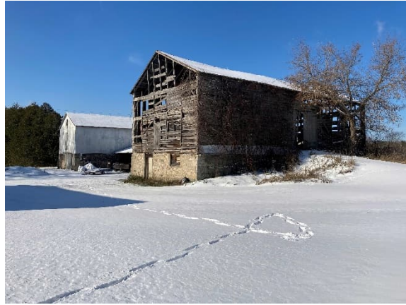
Plate 91: North and east elevations of north barn
